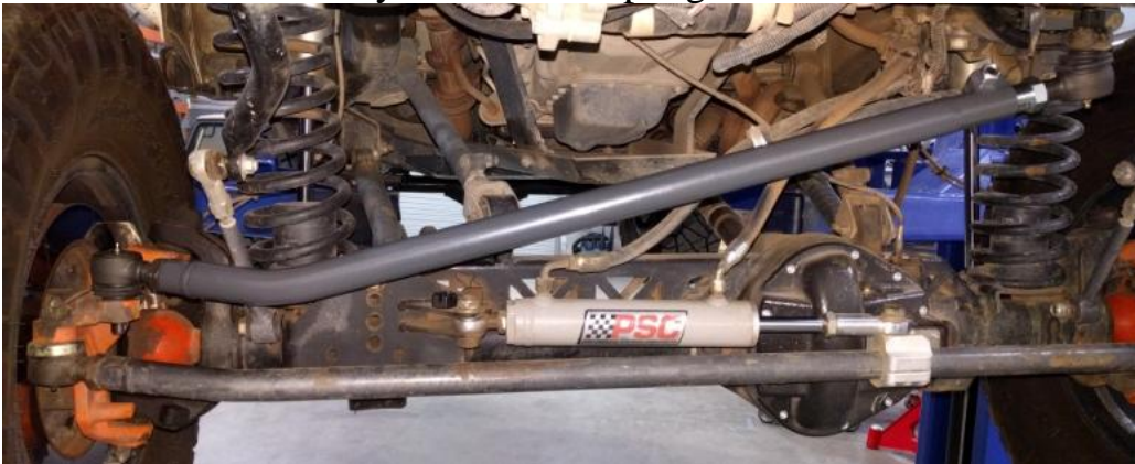
Figure 7. INCORRECT Orientation of Drag Link
