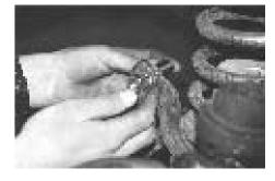
45. Use the pin for leverage with tightening the nut with a 3/4" wrench.
