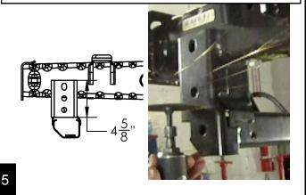
The cross member and support will look like this after cutting. Use a flap disc or grinder disc to make the cut flat.
